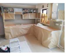
We begin the masking process, All Surfaces are protected from any overspray and ventilation is set up. We begin with a chemical bonding agent and get ready for the first application of colour-matched primer. We air-dry the surface and get ready for the Stone Fleck coating.
